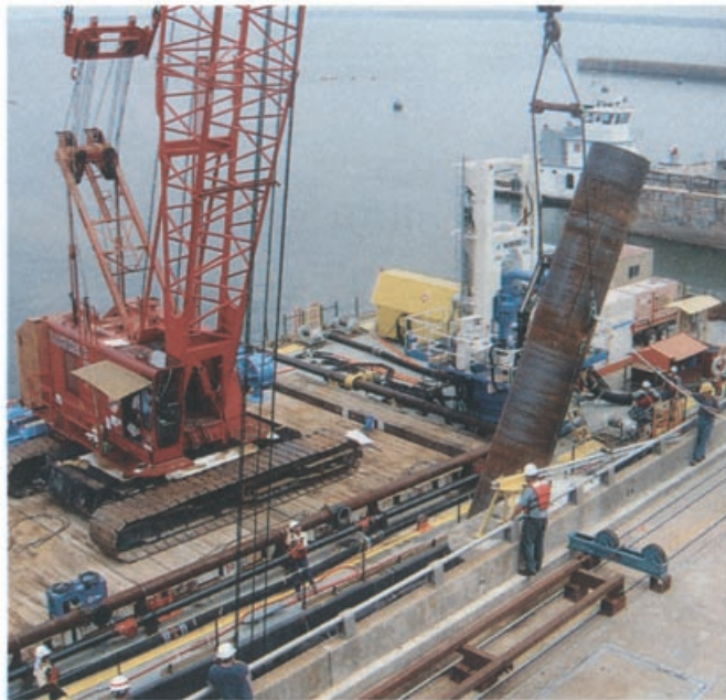
LINING UP Temporary steel casings are used to place piles.
